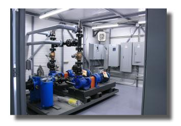
eliminating errors from multiple hand-offs. The *envirosep MPH* is controlled by a non-proprietary, programmable controller, providing the best system operating efficiency. Variable frequency drives may be incorporated with manual or automatic bypasses. The user-friendly, color touch screen operator interface is utilized for simple operation. Our experienced engineering staff are available to assist facility owners or engineers in conceptual development and planning.
