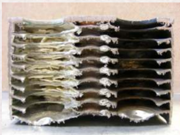
Figure 10. Fouling and clogging of a heat exchanger.
