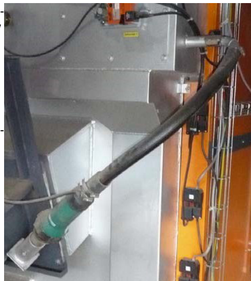
Fig. 6 Automatic ignition (stoker)
