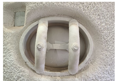
Manway cover prior to adjustment.
