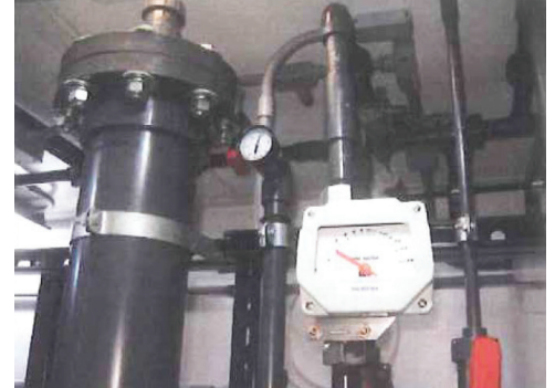
Influent Flow Meter and No. 1 Kinomix™ Proprietary Mixing Reactor Unit.
